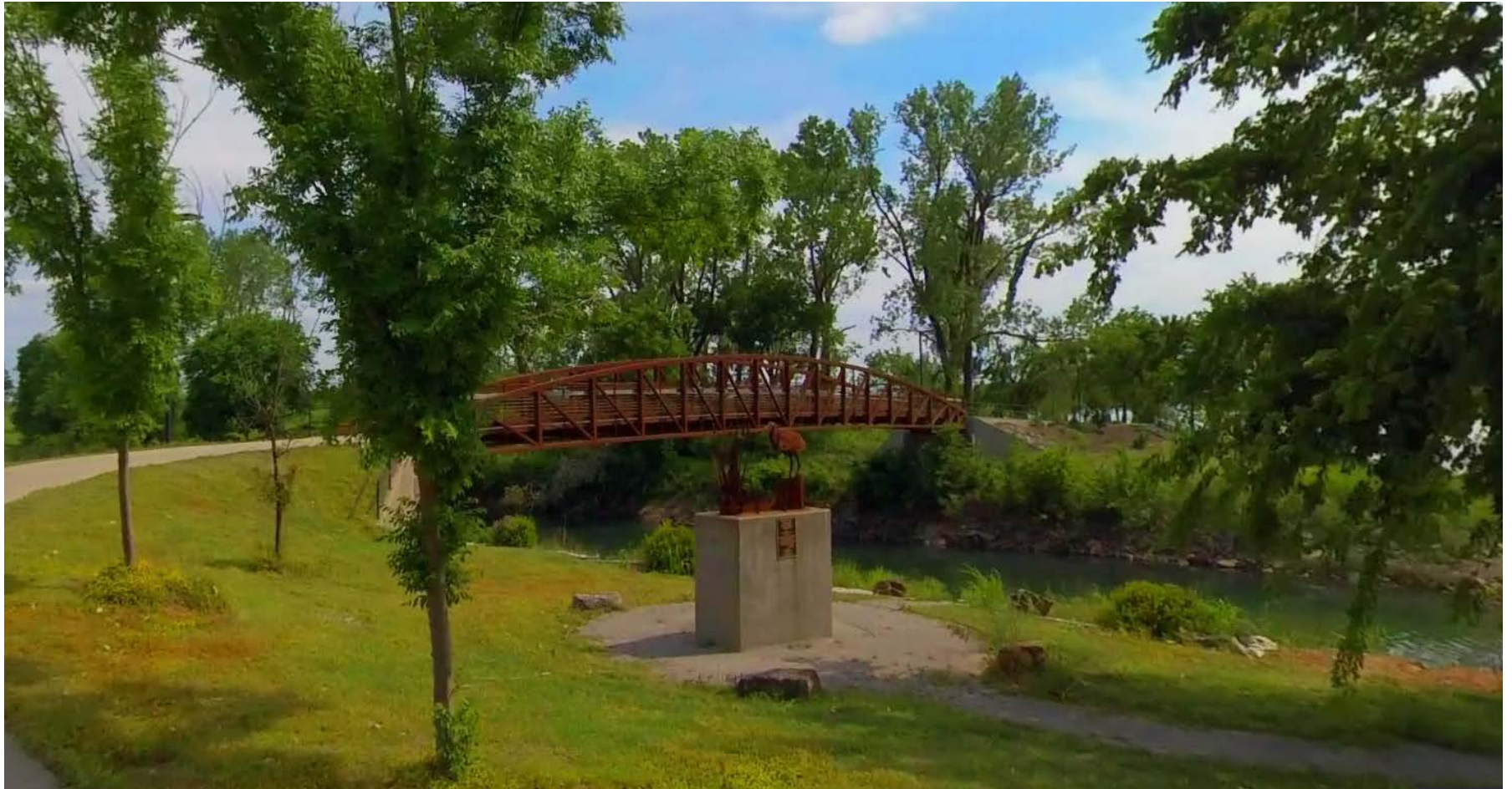
Pedestrian Bridge, Riverfront Drive west of North P Street
